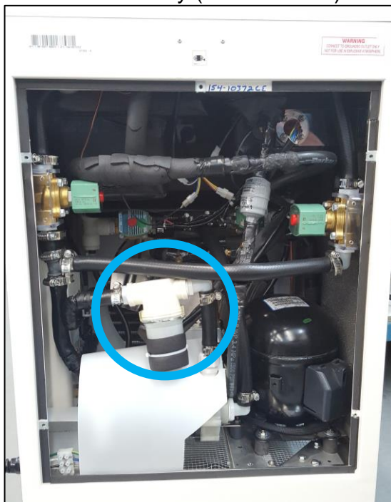
Figure 3-1 Water Filter Assembly
