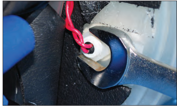
Figure 52 - Step 4 Secure float switch mounting nut
