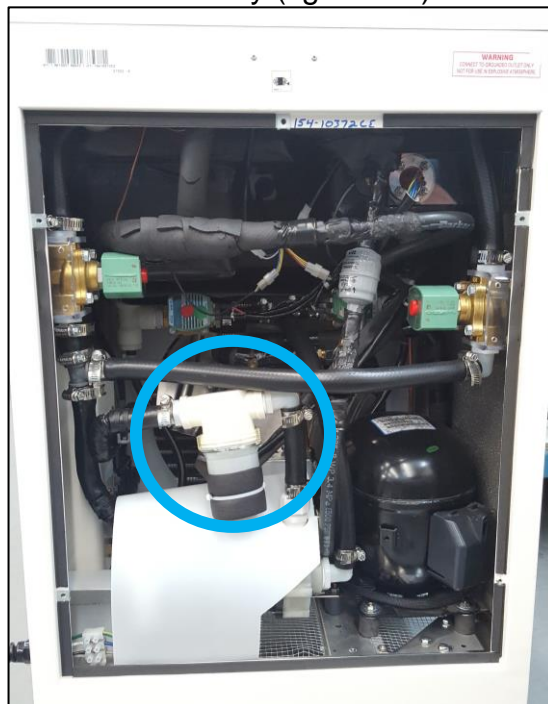
Figure 3-1 Water Filter Assembly
